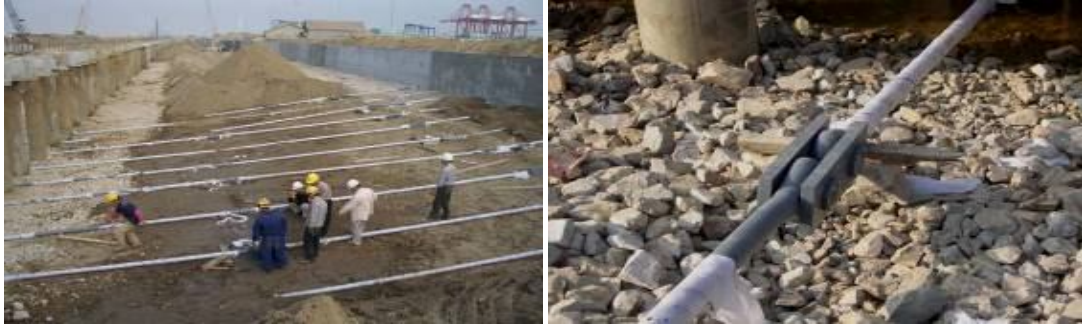
The Qasim port project in Pakistan
